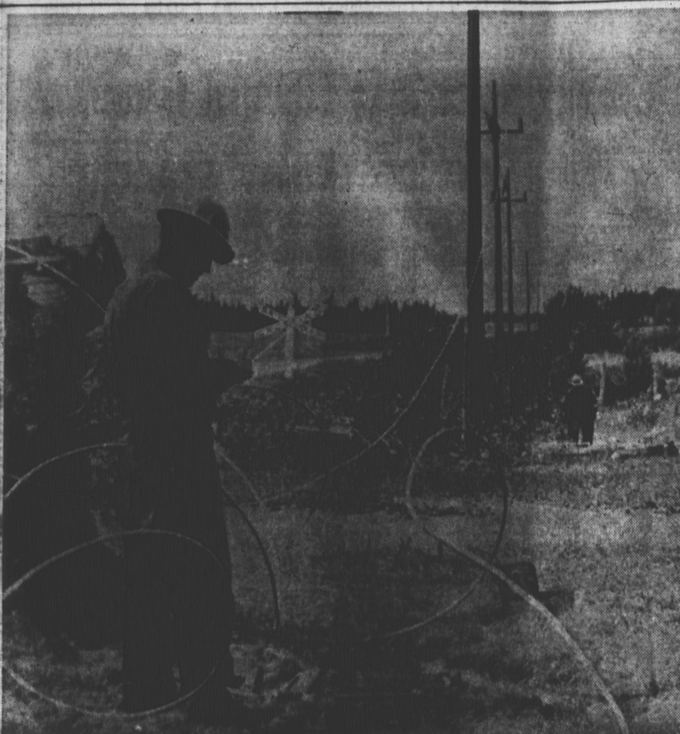
RUNNING POWER LINE TO GEORGETOWN
