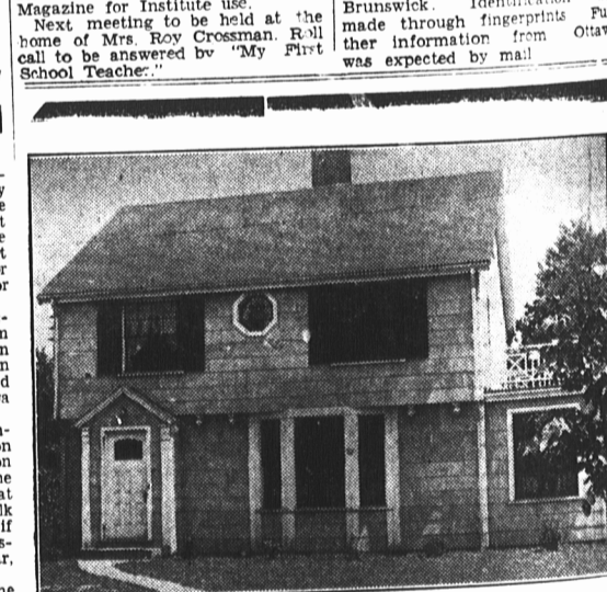
The above residence was recently built for a Charlottetown citizen by MacAulay & Boisner.
