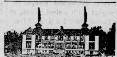
MUSKOKA FREE HOSPITAL FOR CONSUMPTIVES. MAIN BUILDING FOR PATIENTS.
