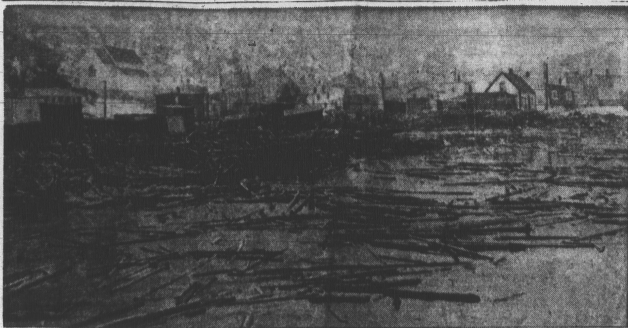
STORM CAUSES DAMAGE IN NFLD.
