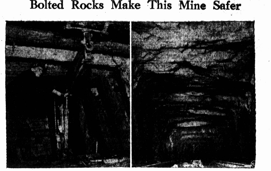
NEW LOOK INSIDE MINES: Old-style support uses timbers (left); new style prevents cave-ins by bolting rock strata of roof together, then cement-coating the whole thing with a spray gun.
