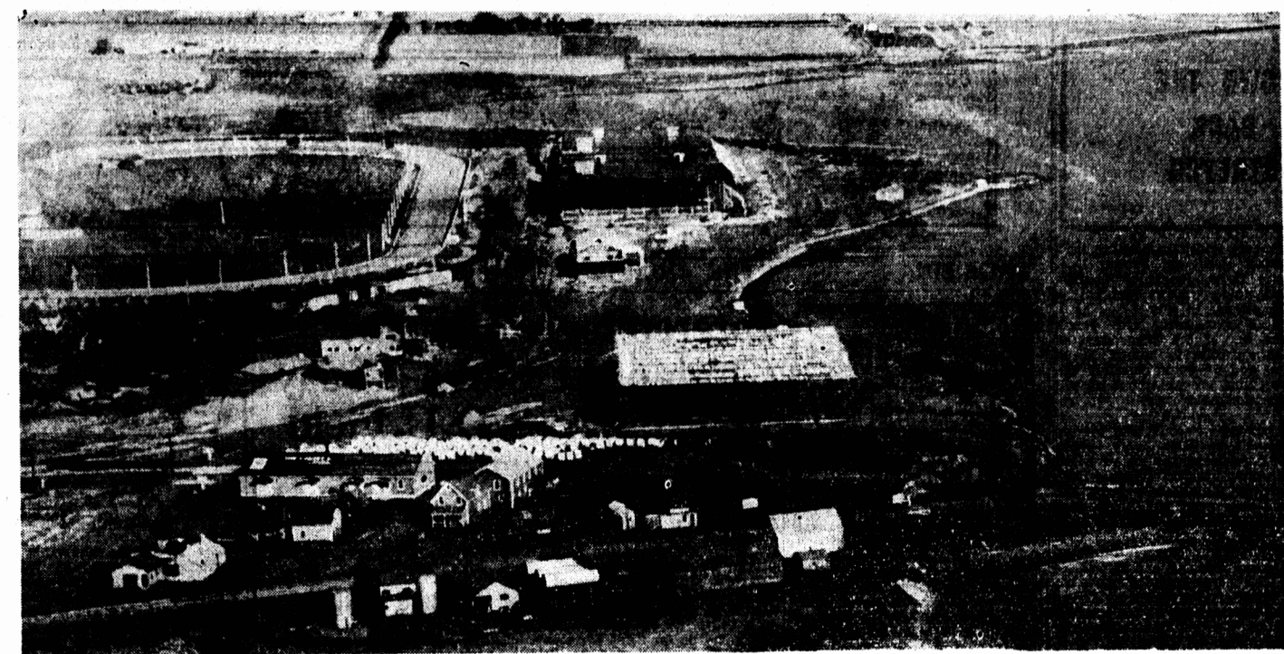
Pictured above is an aerial view of the new industrial development at the east end of the Hillsboro Bridge. The small structure shown centre left, near the race track, is the cement plant of M. F. Schurman which has been producing ready mixed cement since June of this year. The large building in the background is the Island Fertilizer Company plant which will go into production immediately after Christmas. The completion of this structure has been held up due to the shortage of steel necessary to complete the walls. Shown in the centre of the picture, near the fertilizer plant, is the waxing plant of Associated Shippers. This building will be completed in another month. The unfinished structure in the foreground is the new Government Garage which will be completed upon release of the men from the other building projects. —Photo by Paul's Flying Service.
