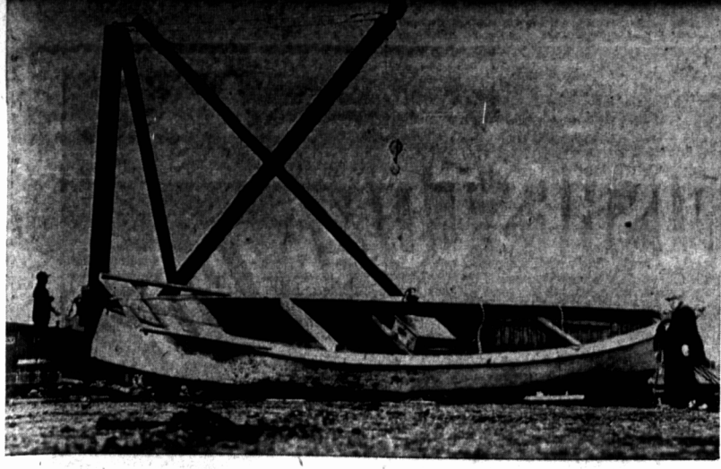
NEW DERRICK FOR OUTHAULING BOATS A large, heavy hoist recently installed on Holman's wharf in Summerside by the Federal Government for the benefit of fishermen and other boat owners, is shown above, being placed in operation Friday for the first time when two large fishing boats were hoisted from the harbor water for winter storage. Photo By Wotman
