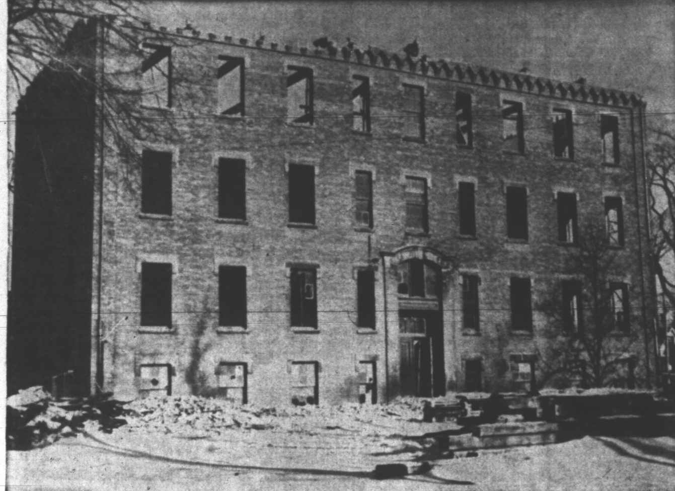
OLD SCHOOL BEING DEMOLISHED
