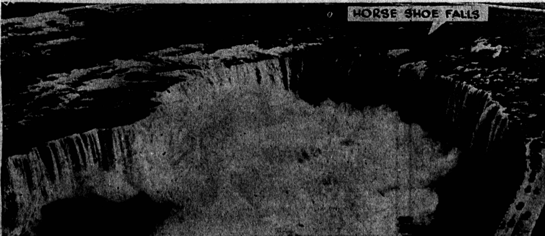
The horseshoe is to be removed from the Canadian Horseshoe Falls. Government plans to spend $700,000 building a series of submerged dams and shearing off shelves on the shoulders of the Falls, to relieve pressure on the centre by forcing more of the water to slop over the Falls at the two flanks. Exposed boulders and shoals are to be removed.
