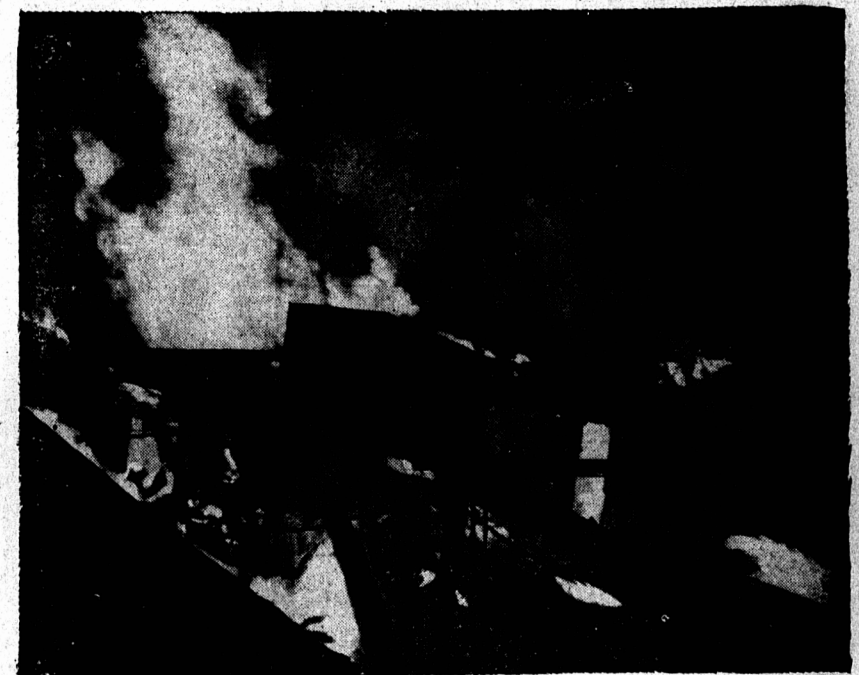
Fifteen hours after flames razed one of Canada's biggest tile works, at Kingston, Ont., firemen still picked their way through the smoking ruins. Fire at its height is shown. Damage was estimated at $30,000; 200 employees are now out of work due to blaze.
