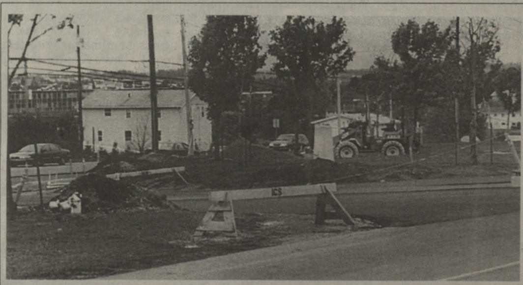
Access continues to be improved upon at UPEI's main entrance.
