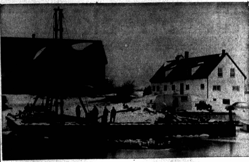
New Wharf At Murray Harbor
