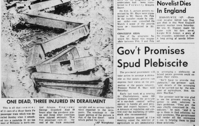
ONE DEAD, THREE INJURED IN DERAILMENT This is all that remains of 11 cars of a 16-car Santa Fe passenger train which was derailed Sunday when it smashed west of a rockpile 15 miles into Williams in northern Arizona. Engineers reported that the train was upright and no serious injuries were reported to the occupants. The wreckage in the upper portion of the picture is a resolution passed at the meeting asked the minister of agriculture to act immediately (AP Wirephoto)
