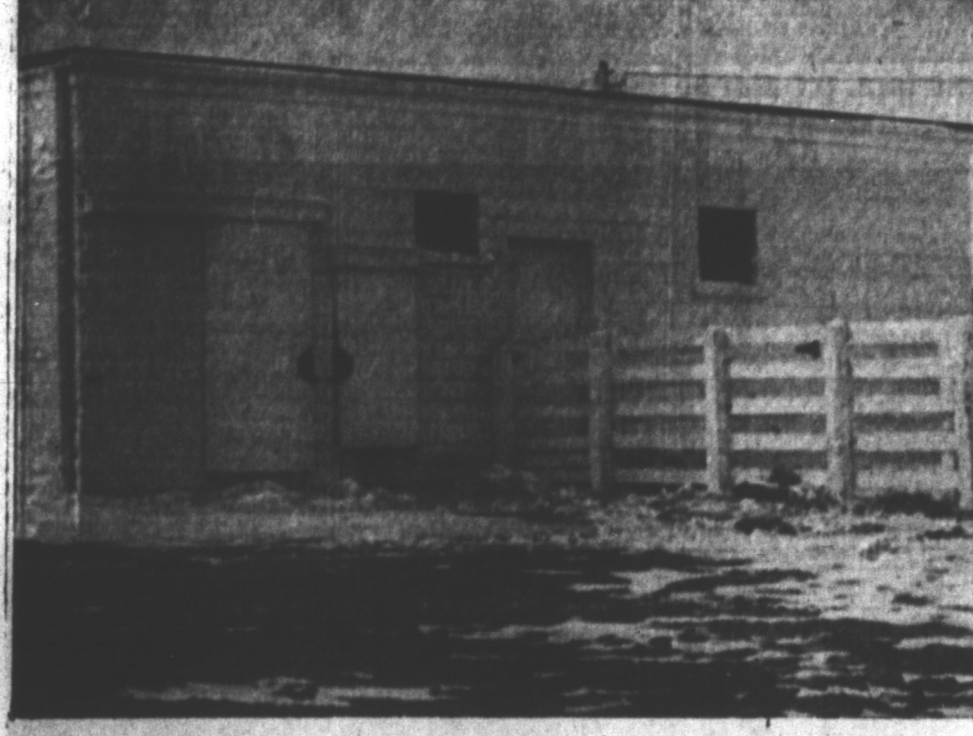
ERECTION OF ABATOIR WAS AN OTHER ST. ELEANORS ACHIEVEMENT.
