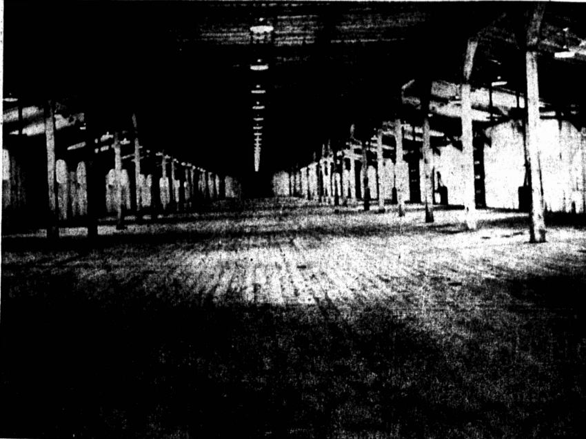
Mr. J. Watson MacNaught, M.P., announced yesterday that permission had been received during the day to begin using the newly constructed warehouse located on the west side of the Marine Wharf in Summerside for the storage of potatoes and shippers said last evening that trucks will begin hauling to this new shed today. The early use of this warehouse was made possible through the co-operation of the contractor, J. P. Porter and Co., the Department of Public Works and the Department of Transport. This announcement will be received with much pleasure by shippers and producers alike and is of special timely interest to farmers who have potatoes stored in outside buildings where the risk of frost is great. The interior of this large frostproof warehouse is shown in the photo above. (Photo by Wotton)
