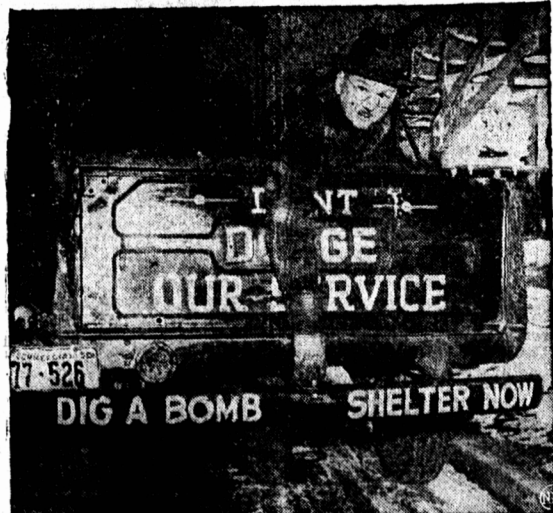
GOT YOUR BOMB SHELTER? — Charles Schuling is doing his bit to persuade Des Moines, Ia., citizens to build their own private bomb shelters. Schuling points to an advertising slogan painted on the bumper of his truck. P.S. He's head of a firm that rents out excavating equipment.
