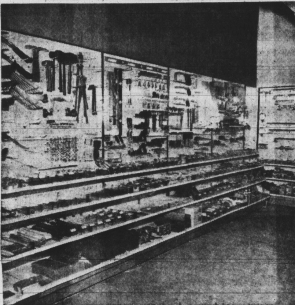
HARDWARE DEPARTMENT, THIRD FLOOR
