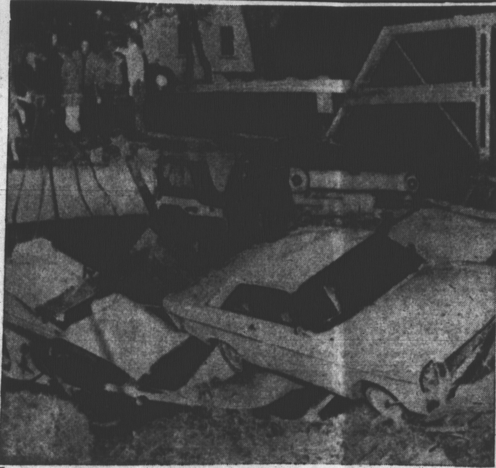
CAR COLLAPSES BRIDGE
