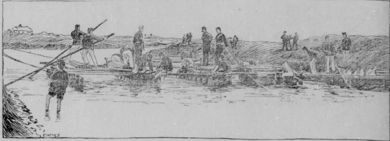
HOW THE ENGINEERS BRIDGED OVER THE TUGELA—COLONIAL TROOPS MAKING A PONTOON BRIDGE.
