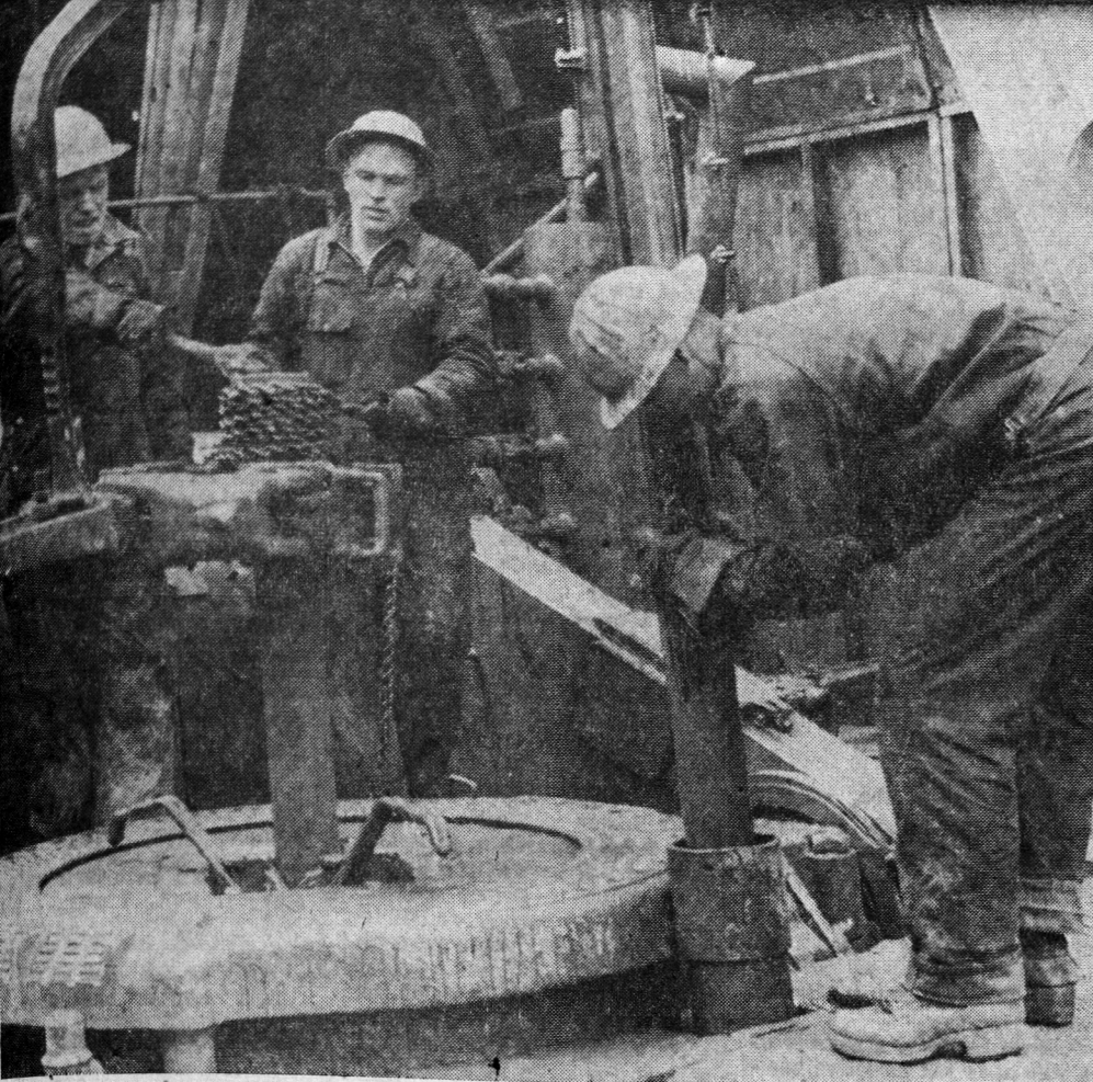
FAST WORKING drill crews are seen adding another 30-foot section of drill pipe at the Imperial Oil drill site at Wellington yesterday where the drill had reached a depth of about 8,700 feet without yet finding oil or natural gas.
