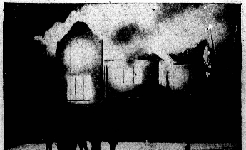
Firemen at Hanover, Ont., found the fire hydrant frozen when one of the town's two public schools burned at 3 a.m. They built a fire and used gasoline torches to thaw hydrant out. Here early spectators stand helpless. School was burned down.
