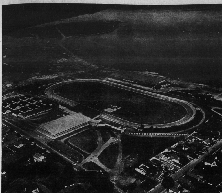
EXHIBITION GROUNDS READY FOR THOUSANDS OF VISITORS AND THE ERECTION OF MIDWAY ALL ROADS LEAD TO CITY FOR OLD HOME WEEK
