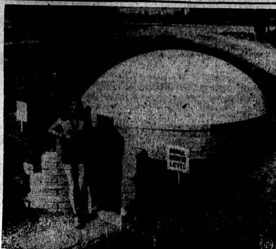
FAMILY FOXHOLE —Latest entry in the parade of home bomb shelters is this dome-roofed, concrete structure, which San Francisco builders say can be installed in your back yard for $1250. The 12½-ton house sleeps six comfortably or 20 in an emergency. When not in use as protection against aerial attacks, it doubles as utility room or guest house. The 14-inch-thick dome and eight-inch walls should be adequate protection from the weather.
