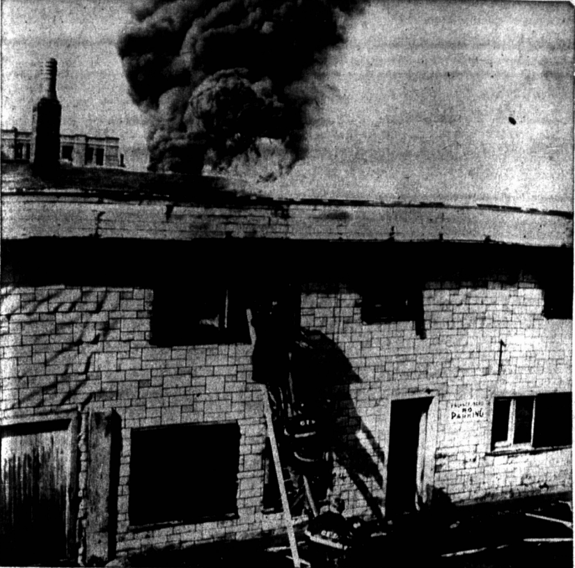
FIREMEN DIRECT A HOSE INTO THE BLAZE
