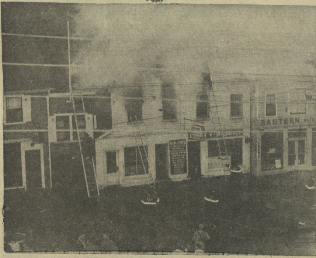
CITY firemen prevented a fire at this three-story wooden building on Gt. George Street Tuesday evening, but a second
