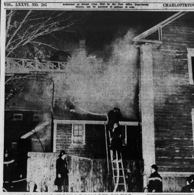
VACANT BUILDING DAMAGED BY FIRE
