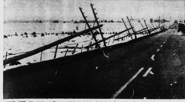
SCENES LIKE this were encountered G of Friday by telephone company linemen in a few areas as the result of Thursday night's ice storm and strong winds. Those poles were on the road north of Montague along Simon Nicholson's farm. Despite the poles being down, most of the heavy load of wires carried appeared to have been unbroken, however.
