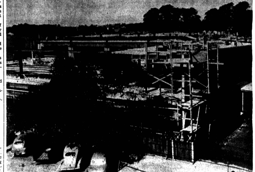
Satisfactory progress is indicated in the erection of the new T. Eaton Co. Limited store on Kent Street (above) scheduled for opening early in the new year. (Garnham Photo Studio).
