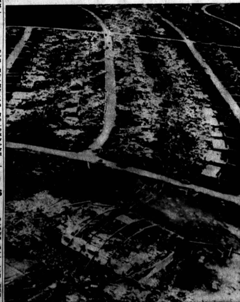
KANSAS CITY—This low level tornado through the suburban Ruskin Heights residential area. In foreground are the ruins of a
