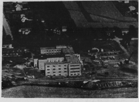
T. ST. MARY'S MOTHER HOUSE TO BE COMPLETED THIS YEAR CONSTRUCTION HITS $641,000
