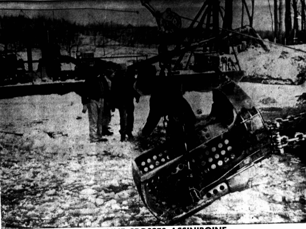
PIPELINE CROSSES ASSINIBOINE
