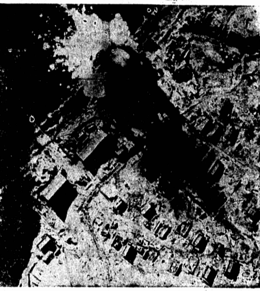
Smack in the middle of Jap installations on Kiska Harbor lands an American bomb. U. S. warplanes from nearby Alaskan bases have blasted these buildings and an uncompleted airfield with raids averaging 100 a month. Continuously here since last June, Japs have had a year to dig in and fortify their positions.
